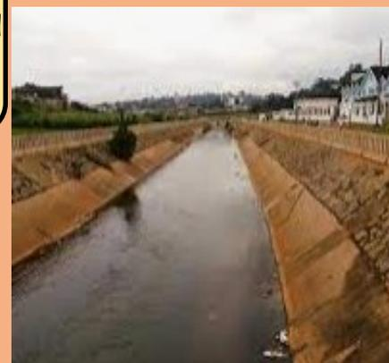
Diversion canals are channels that are man made to redirect and divert water away from certain areas. Flood planes are large open areas designed to allow water to collect instead of flooding houses and urban areas or damaging farm land.
